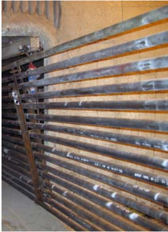
Superheater tubes overlaid with Colmonoy 88
